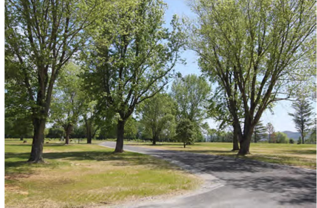
Paving completed at Shawnee State Park
