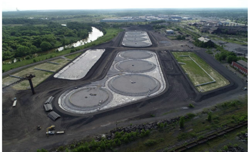
Aerial view of GeoPool construction progress; facing east; June 2024
