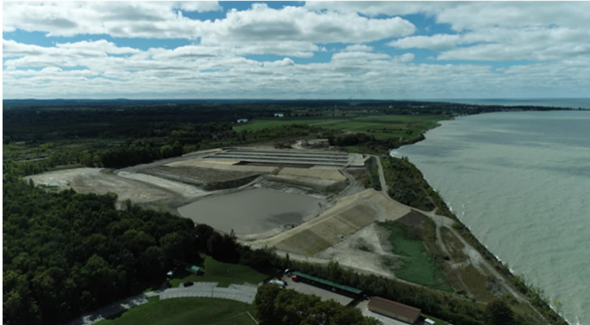
Fairport Harbor, September 2022, Construction in Progress
