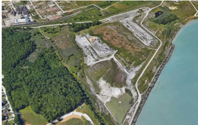
View of Fairport Harbor Site Before Construction
