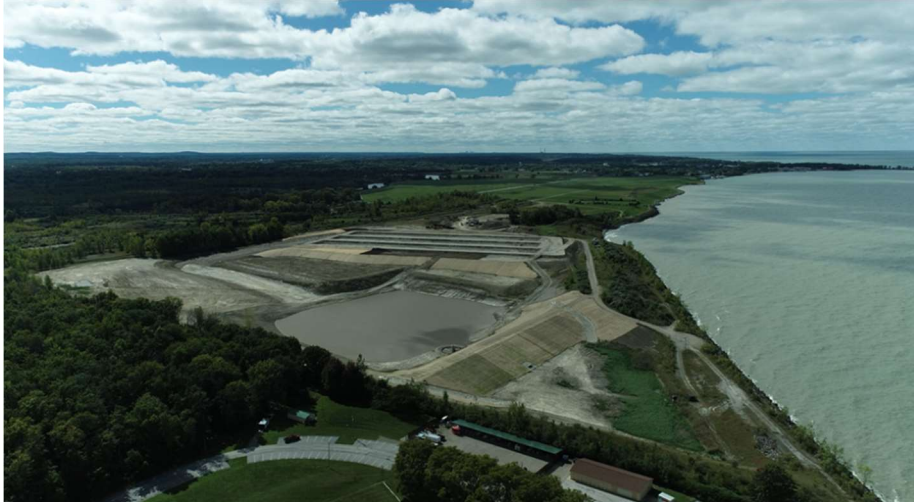
Fairport Harbor, September 2022, Construction in Progress
