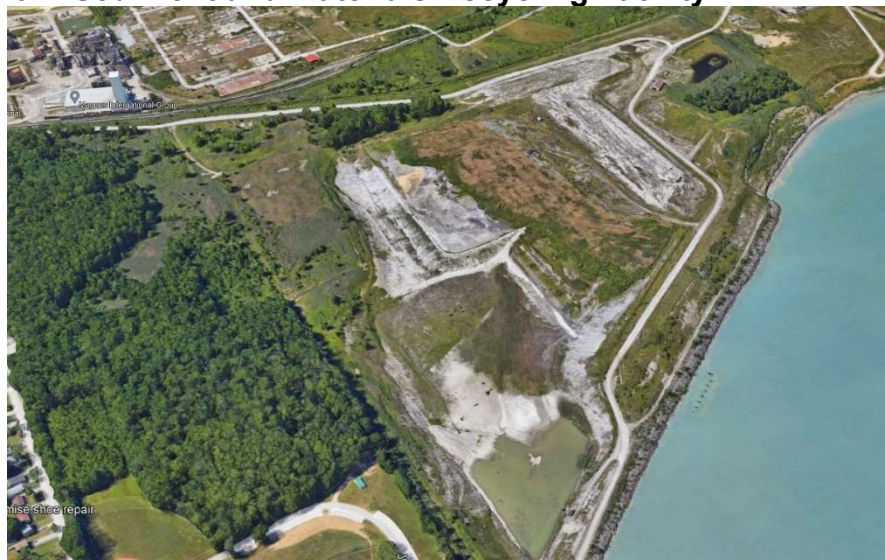
View of Fairport Harbor Site Before Construction
