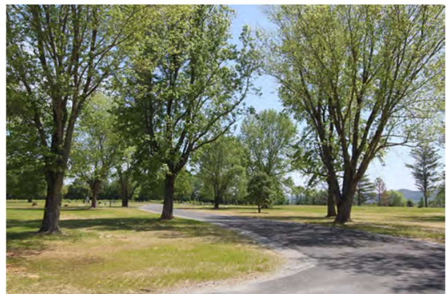
Paving completed at Shawnee State Park
